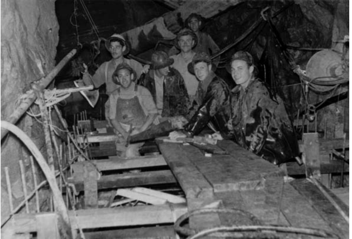
Celedonio Moreno Tejada worked in heavy construction in Melbourne.
