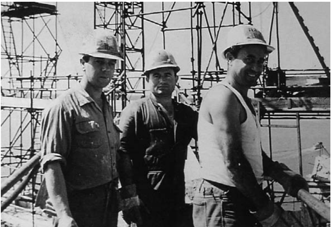
Julian Oriñuela, at left, working in construction on the Sydney Opera House.
