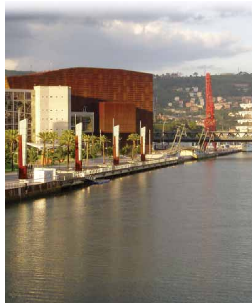
Euskalduna Conference Centre and Auditorium, built over the former Euskalduna shipyard. Bilbao.
