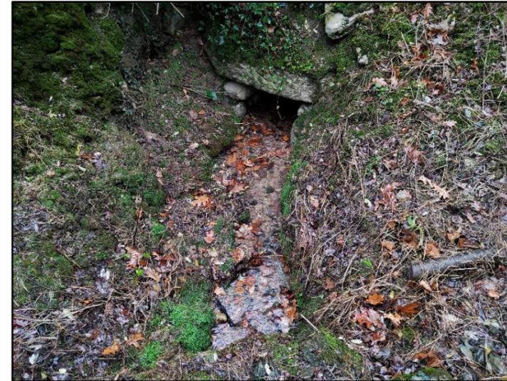
FIGURA 4. EMBOCADURA DEL COLECTOR EXISTENTE. (FUENTE: ESTEYCO)
